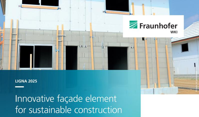
At LIGNA 2025, the Fraunhofer WKI will be presenting an innovative curtain wall element as a sustainable solution for building refurbishment. It uses durable raw materials such as robinia wood and bio-based coatings for less durable types of wood such as spruce and poplar.
